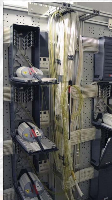
*On each floor there is a cross point that collects and divides each fiber to finally end up in one of the only two cross-fields.*
