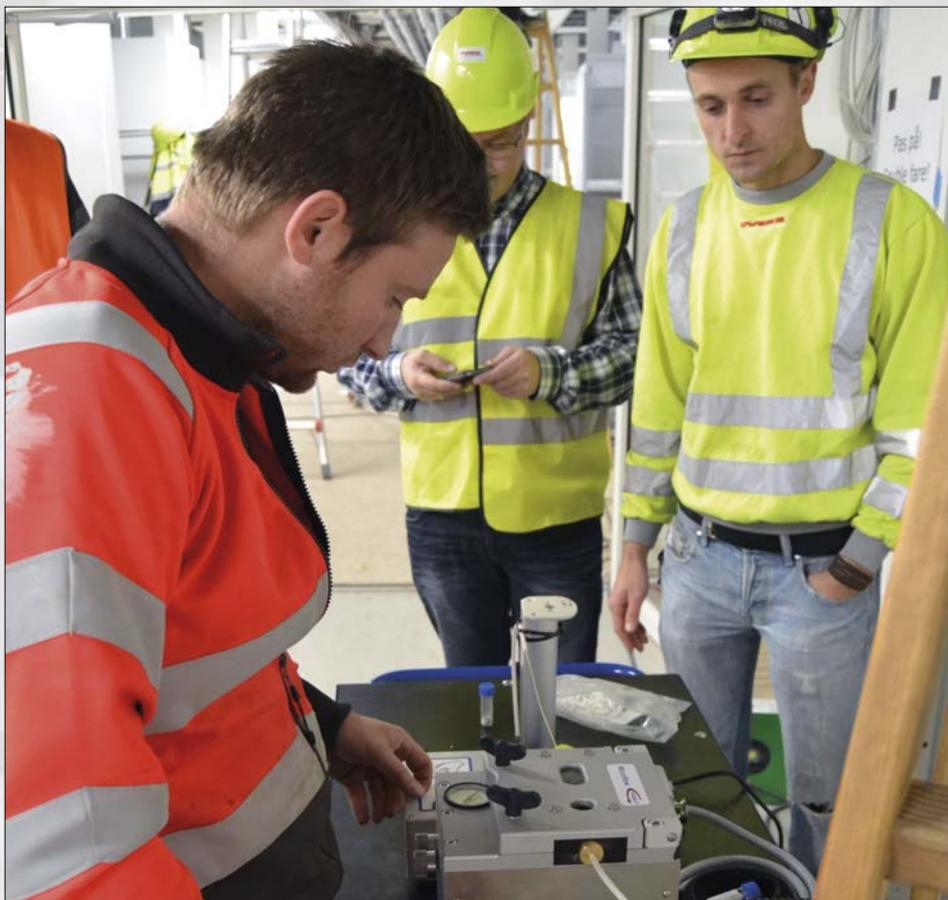
*Chief fitter Jesper Bolding is guiding the technician who is blowing a few hundred meters fiber into the already vastness of Emtelle multi ducts found at the hospital. For the task, one Fremco MicroFlow Touch that really comes to the test with a total of two million meters fiber.*
